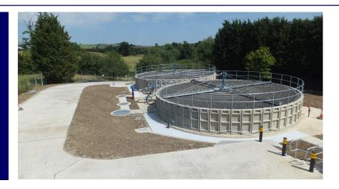
The contract was a consent led upgrade of Cherington Sewage Treatment Works Near Shipston on Stour under Severn Trent's AMP5 non-infrastructure framework. The aim of the scheme was to reduce the ammonia level in the final effluent. The work was carried for Costain as a tier 2 partner under an NEC option C contract.
